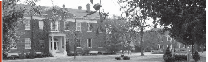
WOHLERS ADMINISTRATION BUILDING
